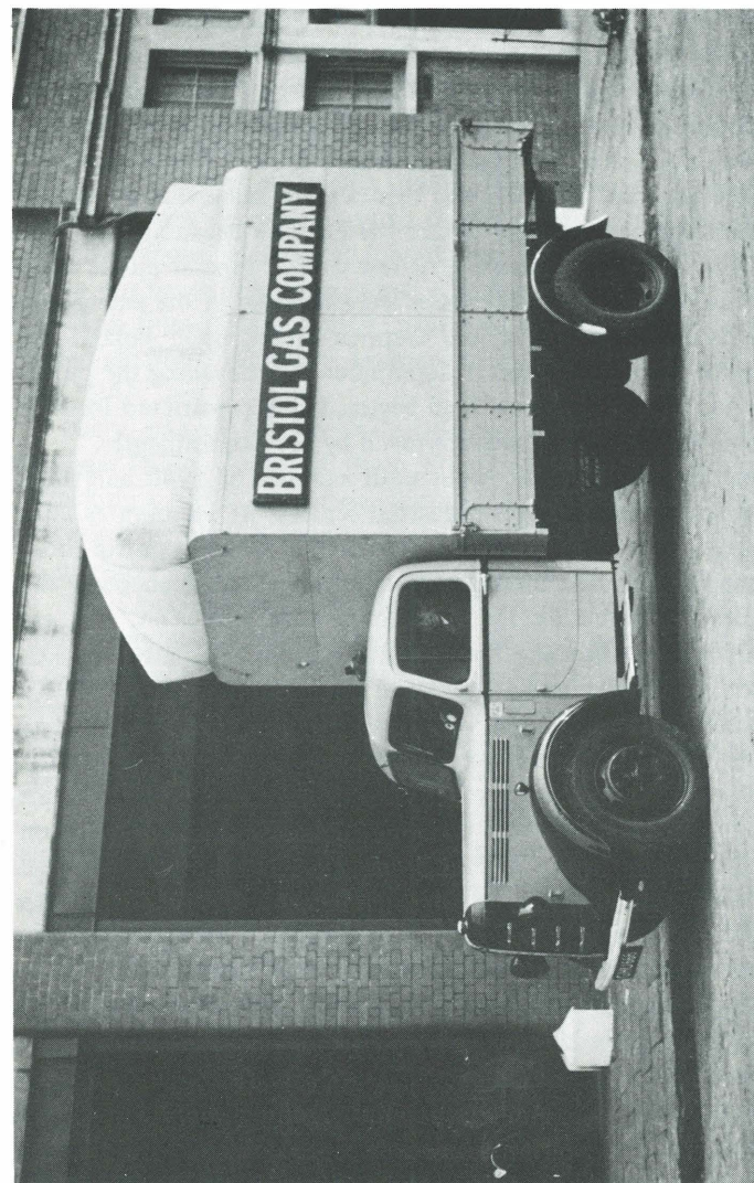
Bristol Gas Company Van — 21 November 1939. A Bedford lorry adapted to gas propulsion seen in Barton Street. 15 miles was possible with this gas bag inflated with 250 cu. ft. Reece Winstone .
